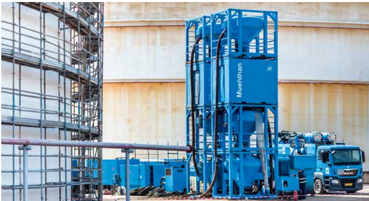
Blasting work on storage tank
