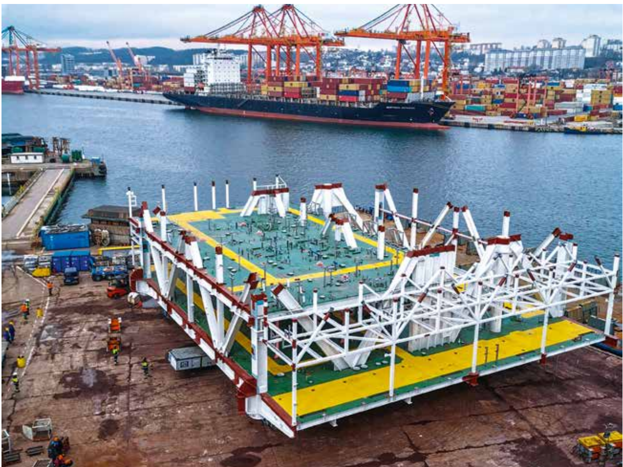
Surface protection work on a module for an oil rig
