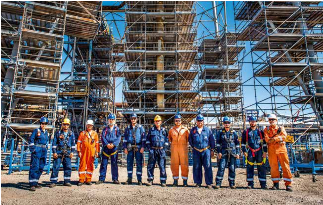
Scaffolding work in Greece
