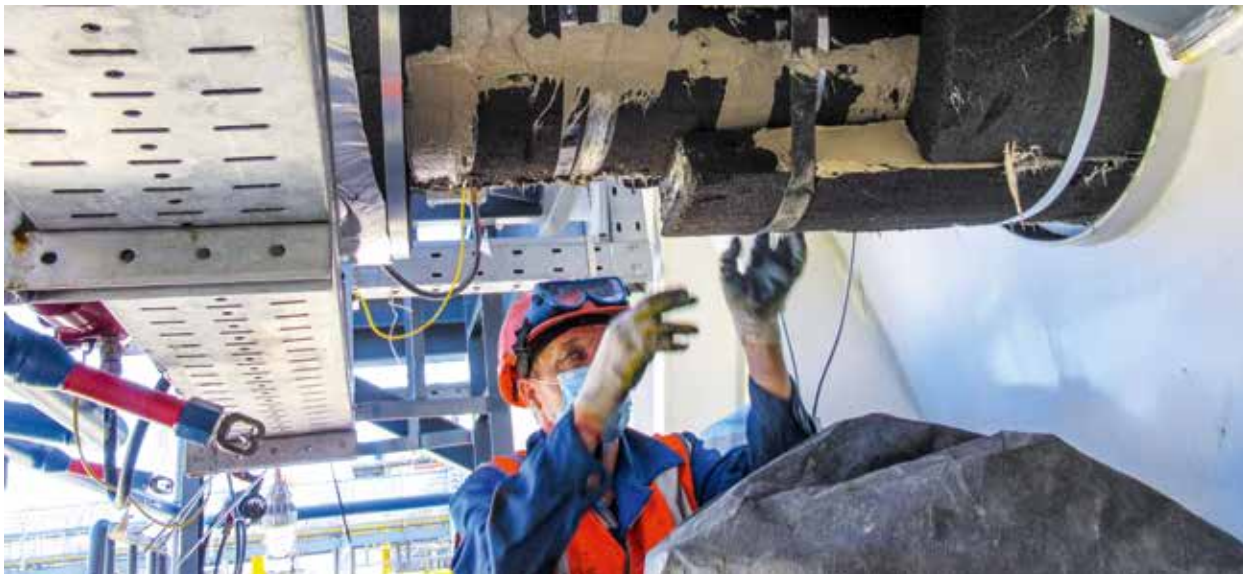
Insulation work on a gas liquefaction station in Russia
