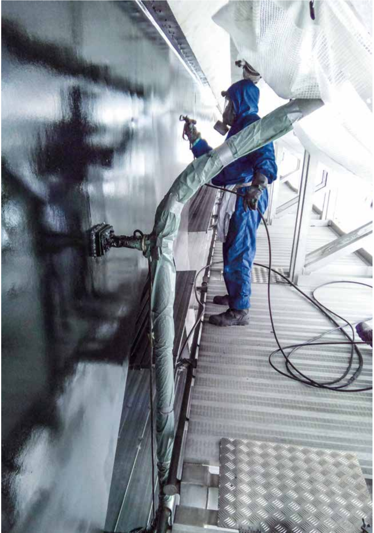
Application of surface protection on the Øresund Bridge in Denmark
