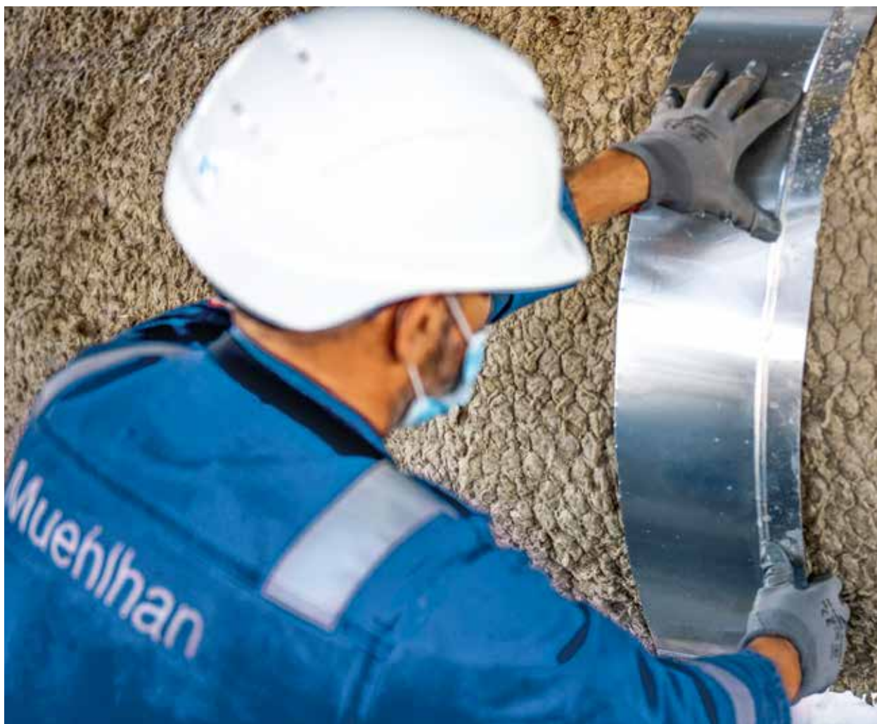
Applying insulation to a pipeline in a refinery
